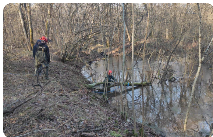
Chantier mare-Marigny-les-Usages © N.Déjean
